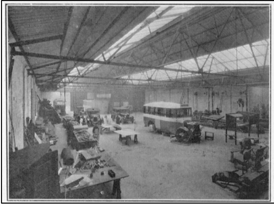
C. 1935 – Jackson’s new workshop at Pittencrieff Street
