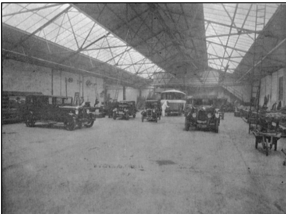
Workshop with the office up stairs on back wall
