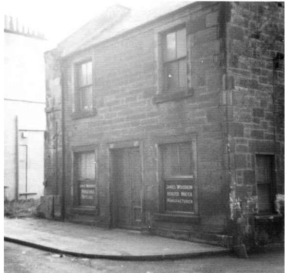
C. 1950 – Woodrow's Office Building at Rolland Street
