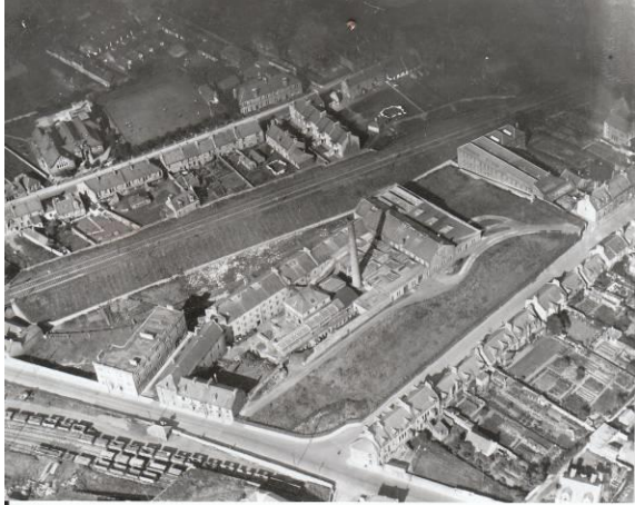
Aerial photograph of Baldrige Works c. 1938
