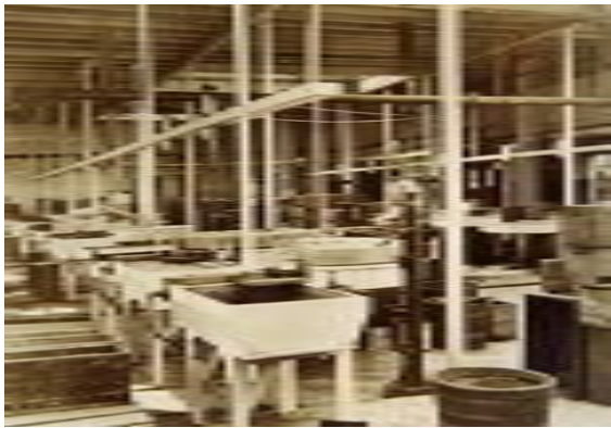
The bottle washing sinks and drying tables
