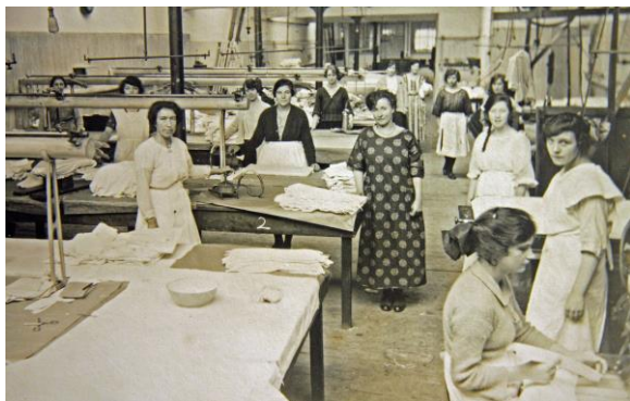
Finishing Ladies at Westfield Laundry c. 1930
