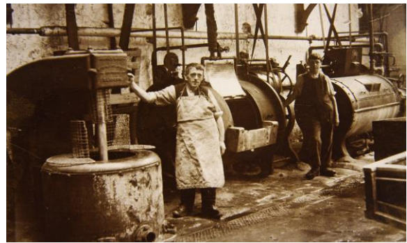
Early belt driven washing machines at Westfield Laundry c. 1910
